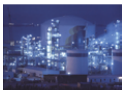
Refinery and petrochemicals
